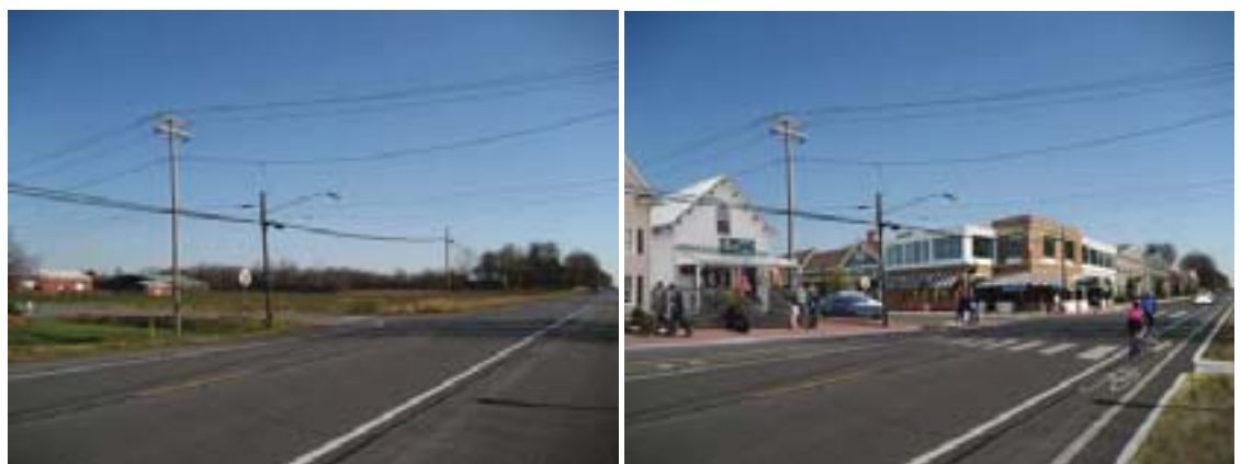
CICERO CENTER HAMLET (ROUTE 31 AT WHITING ROAD)
