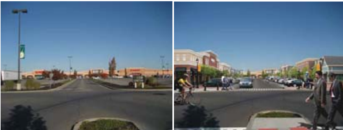
INFILL DEVELOPMENT AT AN EXISTING COMMERCIAL PLAZA (COR CENTER ENTRANCE FROM ROUTE 31)
