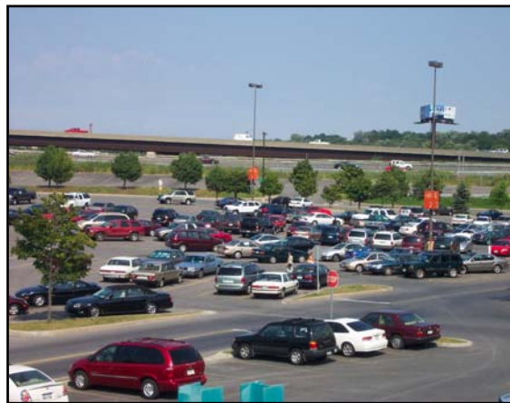
Lack of pedestrian access within parking lots
