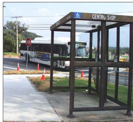
Handicapped accessible transit stop in Onondaga County.
